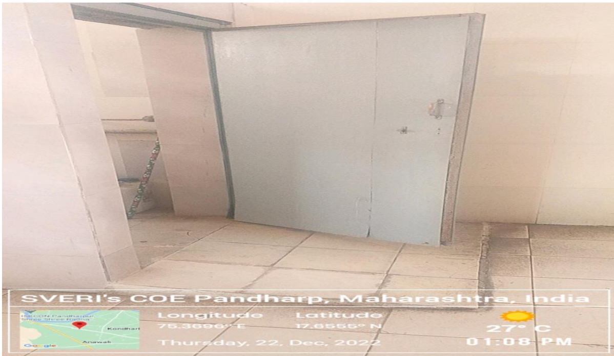
Disabled friendly washrooms
